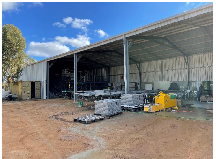
Figure 54: Core processing facilities
